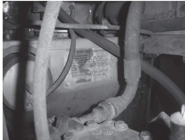
Figure 12-9 Compressor and suction hose or vibrasorber.
