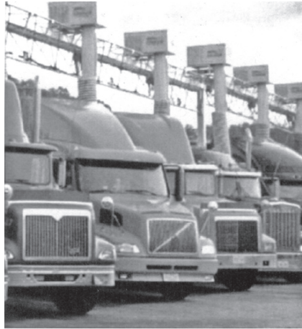
Figure 9-31 Picture of an HVAC stand-alone system contained in a structure above the truck parking space.
